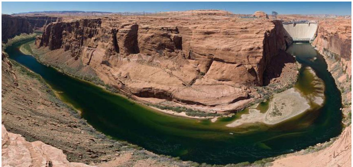
Glen Canyon Dam on the Colorado River © Christine Chessia
