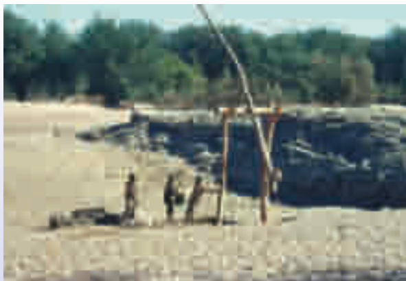
Shaduf used by Topnaar people in the Kuiseb River, Namib Desert, to obtain domestic water and water for their livestock before solar pumps were introduced in the 1980s. The alluvial aquifer depth ranges to about 8m below the surface.
